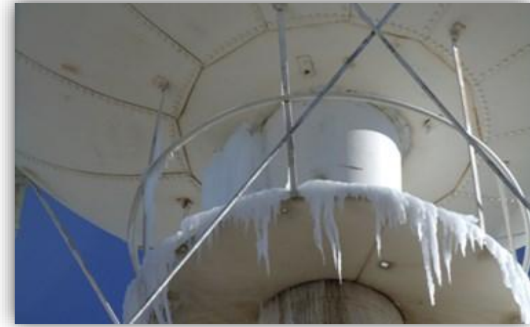
Storage Tank overflow
