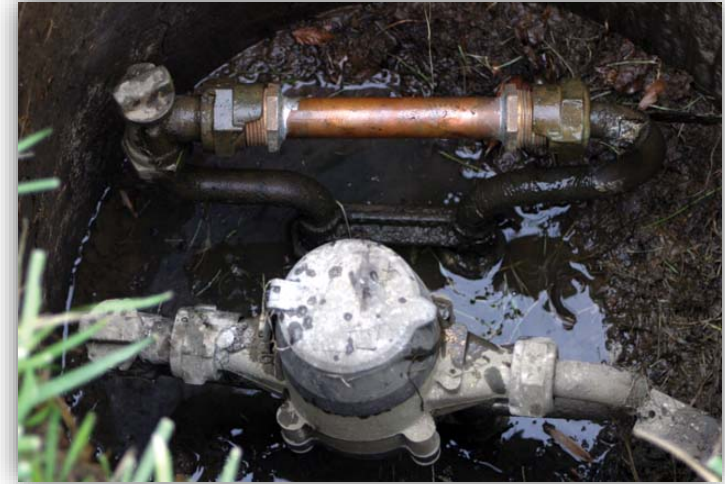
Water meter at top was illegally removed and replaced with a “straight” pipe or “meter jumper”
