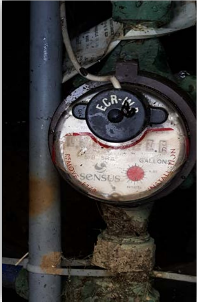
Older 5/8-inch water meter in an outdoor meter pit
